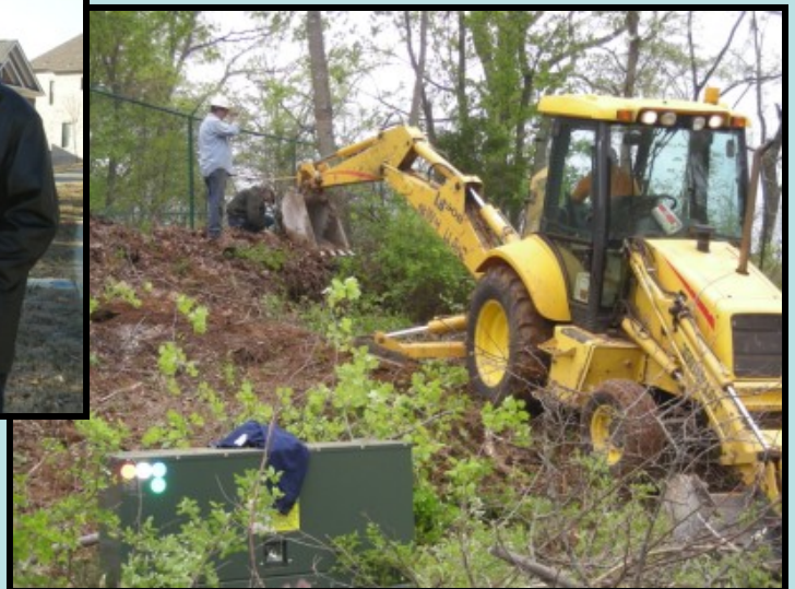
Work started and then stopped
