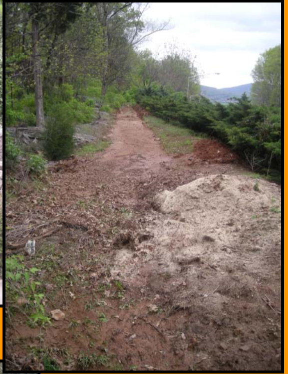
Drainage behind Airport Road berm was improved and berm repaired
