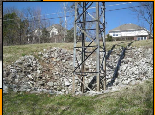
Power tower brush was removed
